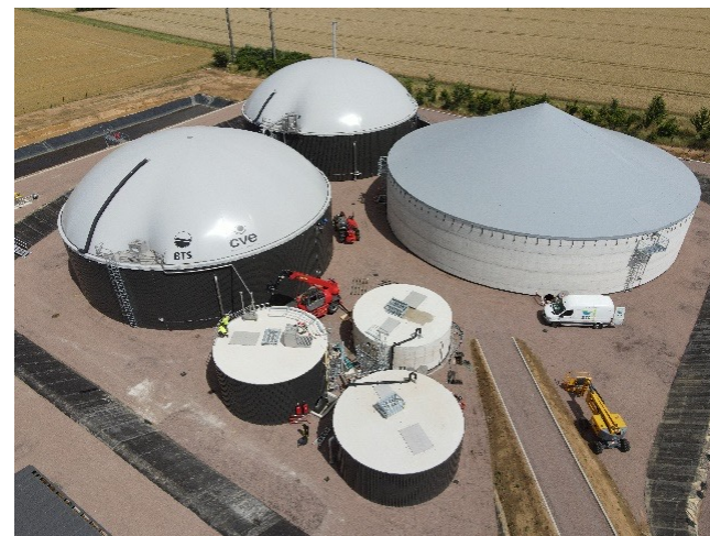
Centrale Equimeth (24 GWh/an)
