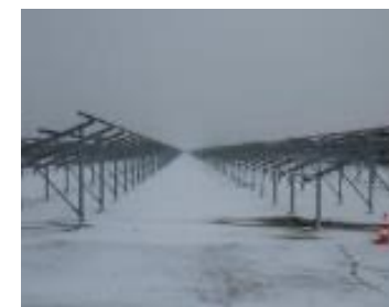
Chantier, Lourches (17 MW)
